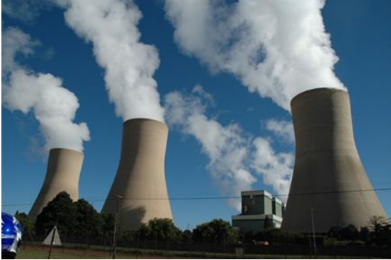
Photo: Duvha power station at Middleburg coal mine in Mpumalanga, South Africa. By Melanie Lamprecht
